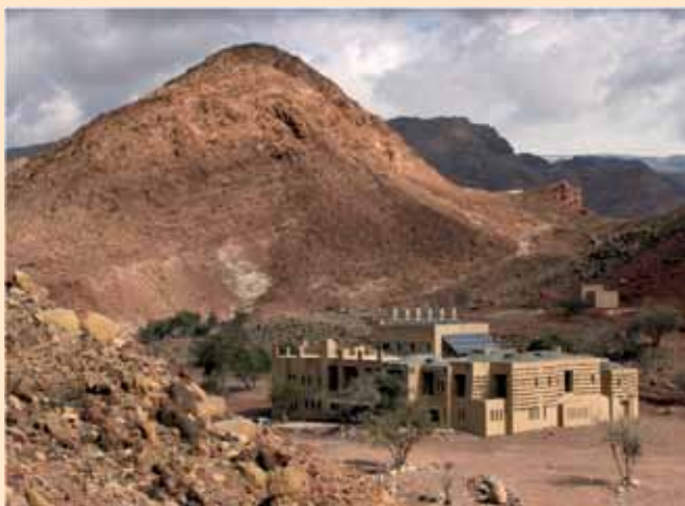
Figure B3: Taking influences from ancient caravanserai and Yemeni architecture, the Feynan Eco-lodge provides 26 rooms, all organically shaped and different in layout. It incorporates several environment-friendly features, including solar power, high insulation and passive ventilation systems and, in the absence of mains electricity, it is lit at night by candle light, which gives a very special atmosphere to the building and creates an unusual attraction for tourists. Feynan Lodge is the first RSCN facility to be outsourced to private sector management
